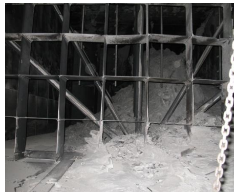
Inlet Turning Vane and Nozzle Pluggage
