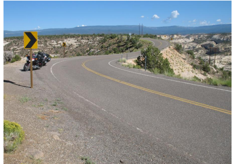
Upcoming Power Plant Driving Deadly if you drop off either edge!
